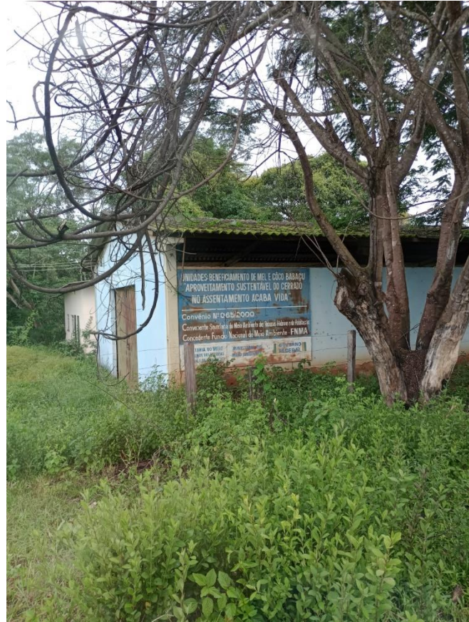
Figure 118. Babaçu coconut factory (abandoned). Source: ECCON Team, site visit, 2023.
